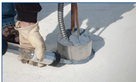
APPLY USING A SAUSAGE GUN
